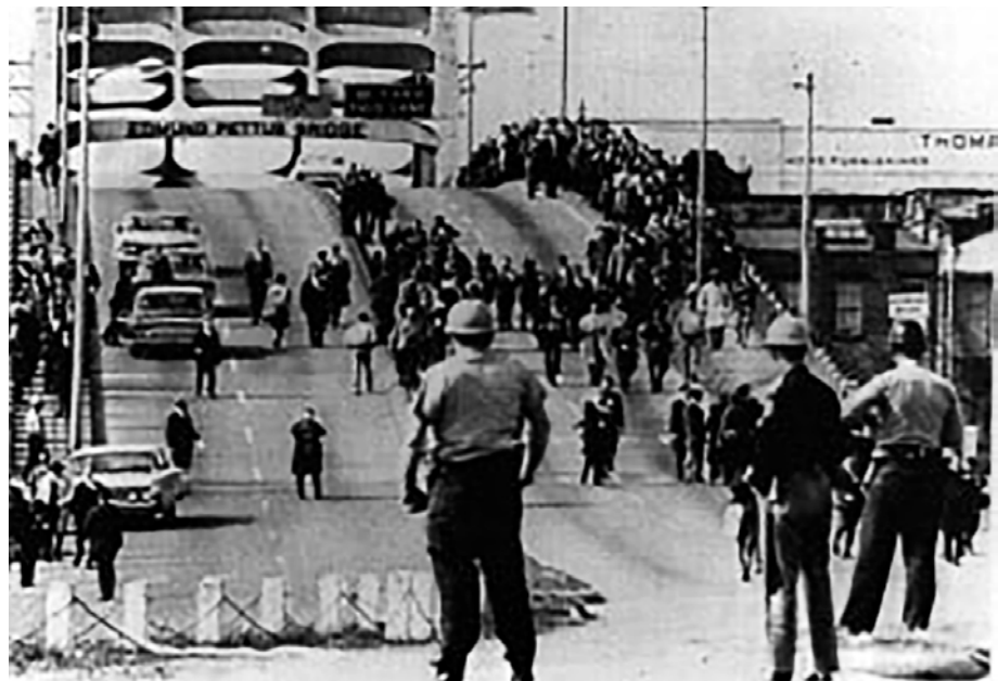
Edmund Pettus Bridge: Bloody Sunday-officers await demonstrators. Photo: U.S. Department of Justice — This is an image of a place or building that is listed on the National Register of Historic Places in the United States of America.
